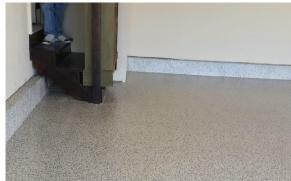
dry ground so it could be installed the same day. After proper prep the base coat of Poly 90 was put down and our Epoxy Color Flakes were added for texture and color. A lunch was taken by the installer then the clear coat was installed. Later that evening the floor was open to light foot traffic!
