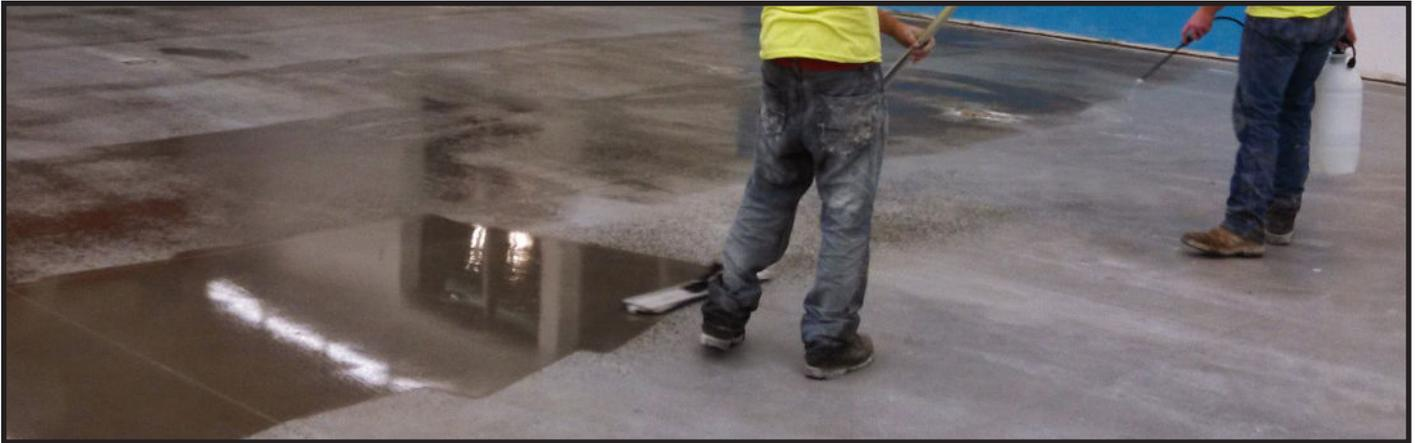
All Crete Densifier is a water based blend of 100% active sodium silicate and silicate polymers that penetrate the surface to increase density, hardness, and strength of the concrete. Those properties reduce dusting, tire marks, and maintenance on the surface. All Crete Densifier penetrates deeply into the surface filling the pores and capillaries of the concrete and reacting with the free lime and calcium carbonate therefore yielding a protected, hardened, and dense floor.
