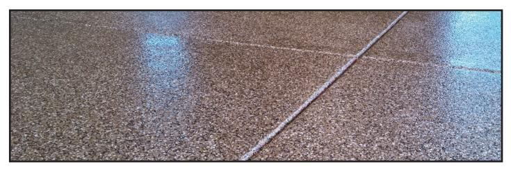
Poly 80 is a two-component Polyaspartic Aliphatic Polyurea utilizing innovative proprietary Nanotechnology. It provides a high gloss clear coating. It's extremely quick curing time provides unmatched labor-saving capabilities above epoxies and polyurethanes. Poly-80 can be used for most types of interior applications over properly prepared surfaces. It's superior penetration and bonding strength can provide years of abrasion, impact, and wear resistance.
